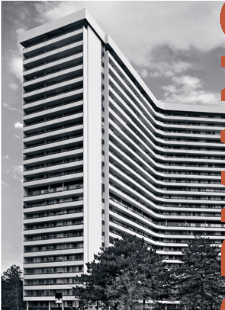
RIDEAU TOWERS III, TORONTO, ON
